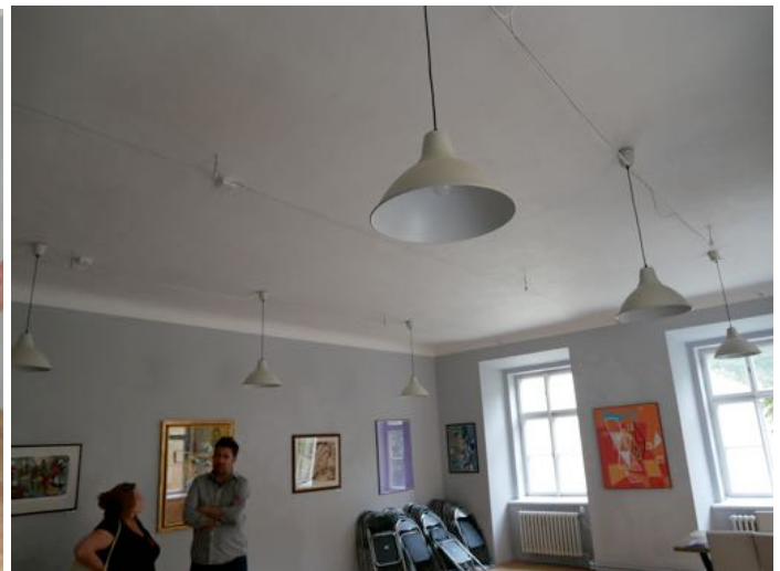
Ceiling with Lights
